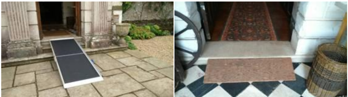
Ramp over 3 steps at front of House and ramp over 1 internal step
