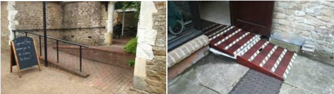
Brick paved ramp to Tea Room and wooden ramp over step in to Tea Room
